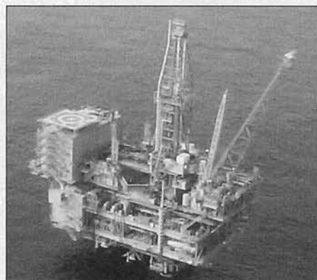
The Jade platform in Zafiro oil field off Equatorial Guinea is the largest fixed production-drilling platform off West Africa (Fig. 1).
